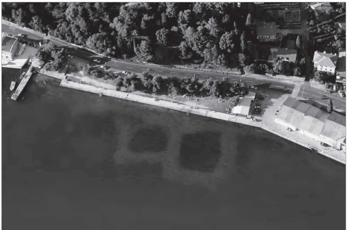
Fig. 2. Aerial photograph of the submerged structure at Fazine near Portorož (photo: Benjamin Jonathan).
